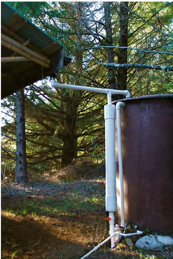
Example of a first flush device (white, vertical PVC pipe, left). Illustration of the working principle of the device (right). Source: DOLMAN & LUNDQUIST (2008).
