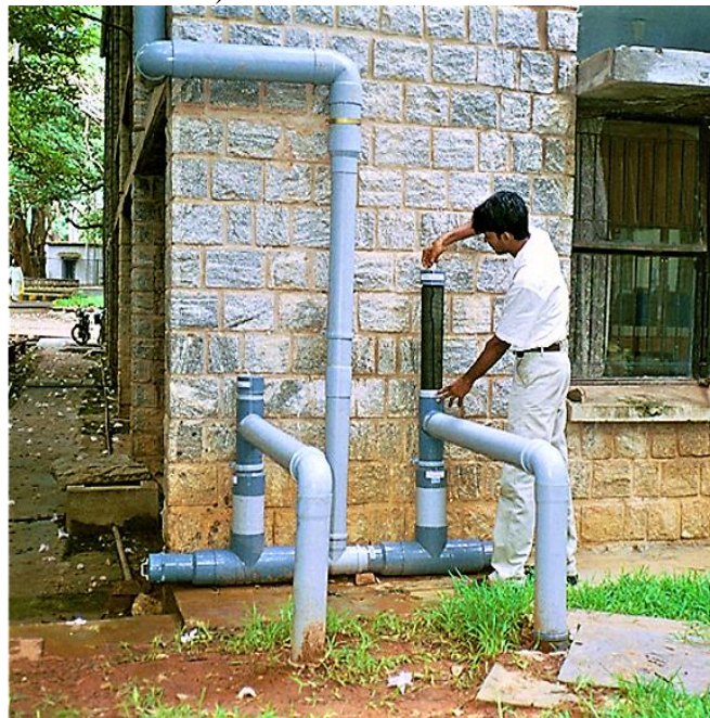
Left: this filter (developed by WISY) fits into a vertical down pipe and acts as both filter and first-flush system. Right: filter cartridge of Pop-up-filter (developed by KSCST) acts as a first-flush separator. Source: CSE (n.y.), KSCST (n.y.)
