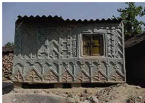
Above ground storage structures
