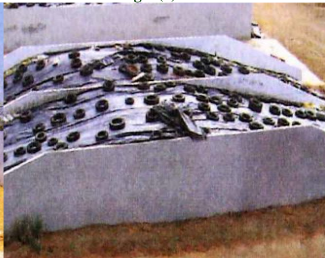
Fig 2(c) Sealed silo
